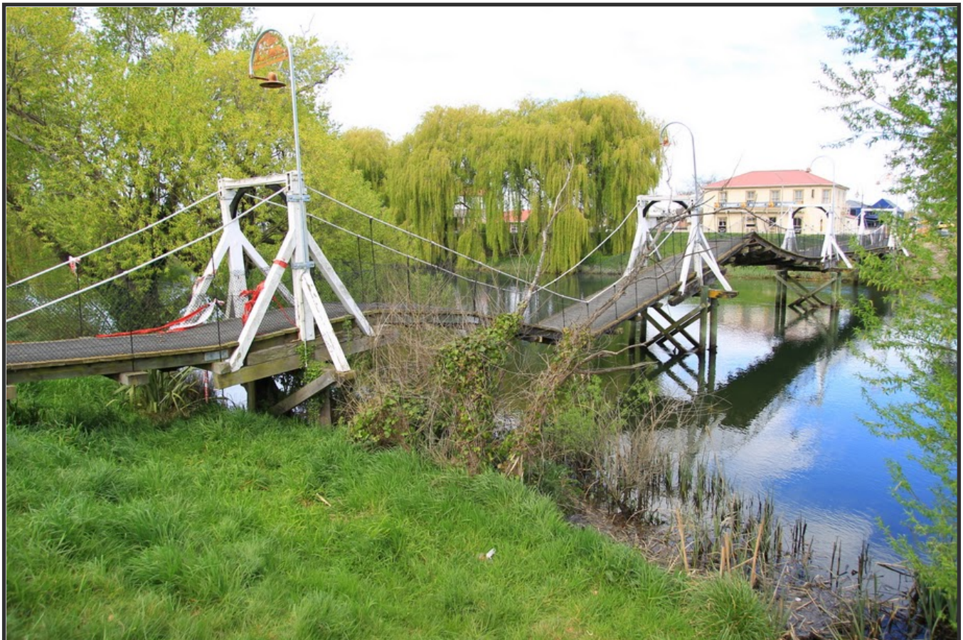
▲ A once serviceable bridge over the River Cam, Kaiapoi, before demolition, September 2011 — ©2011 Ross Becker
